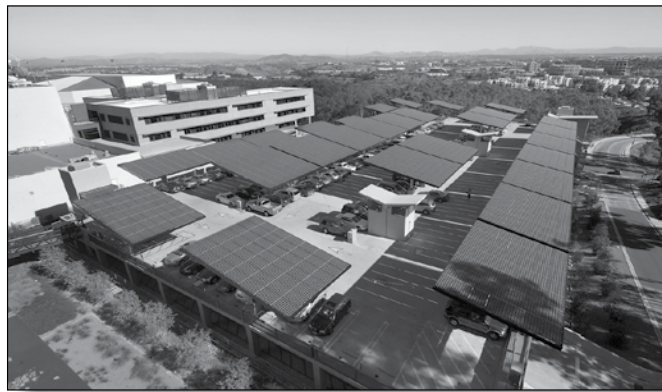
Solar Trees on Hopkins parking structure
